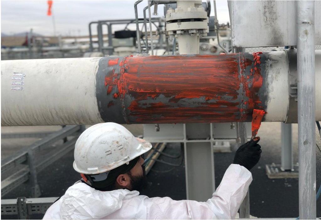
Figure ۶-۲ Apply Epoxy Resin on the pipe surface
