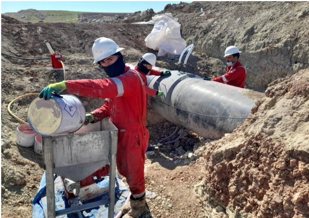
Figure 0-2 Epoxy is pumped into the annular space until it comes out
