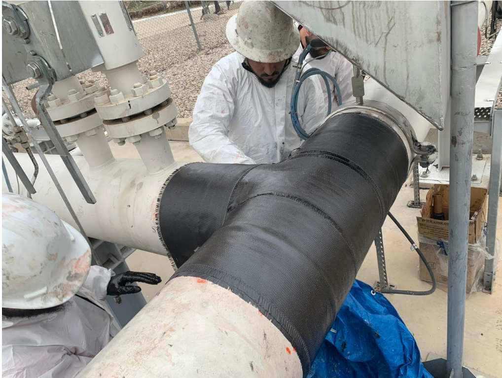
Figure ۶-۵ Apply and Wrapping Fiber Reinforced Polymer on the Pipe
