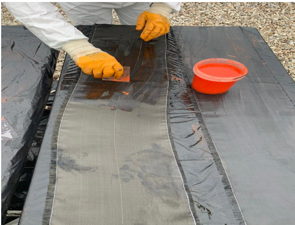
Figure ۶-۲ Apply Epoxy Resin on the Fiber Reinforced Polymer
