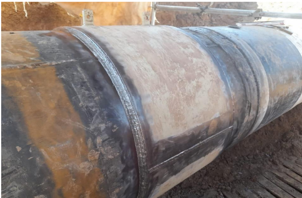
Figure 0-9 Sleeve type B (direct welding)- -36 Inch Kurdistan Pipeline- Erbil
