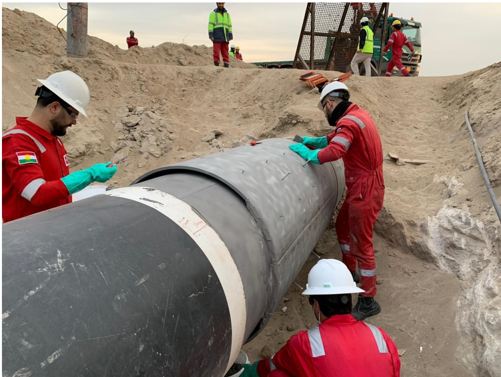
Figure ۵-۱) Type A Sleeve- The gaps at the ends are sealed with quick curing putty
